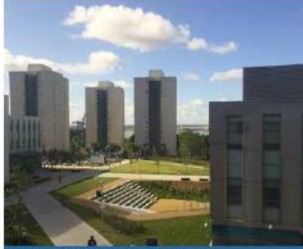
Edge of centre development, Grays
