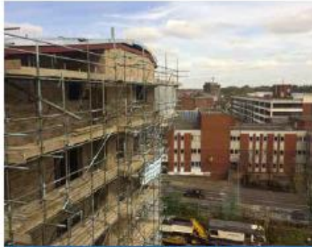
High density residential development at the former Pullman Tavern site in Grays
